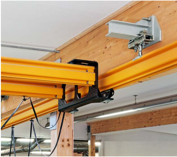
Rear-side anchoring of the support console to the laminated wooden beam.
